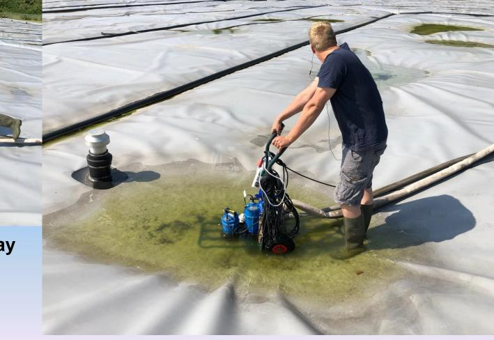
On April 14<sup>th</sup> 2021 we discovered: The floating liner was torn above the top inlet diffusor.
