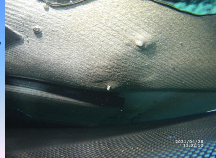
The top diffusor was bend from the weight of the sunken floating liner.
