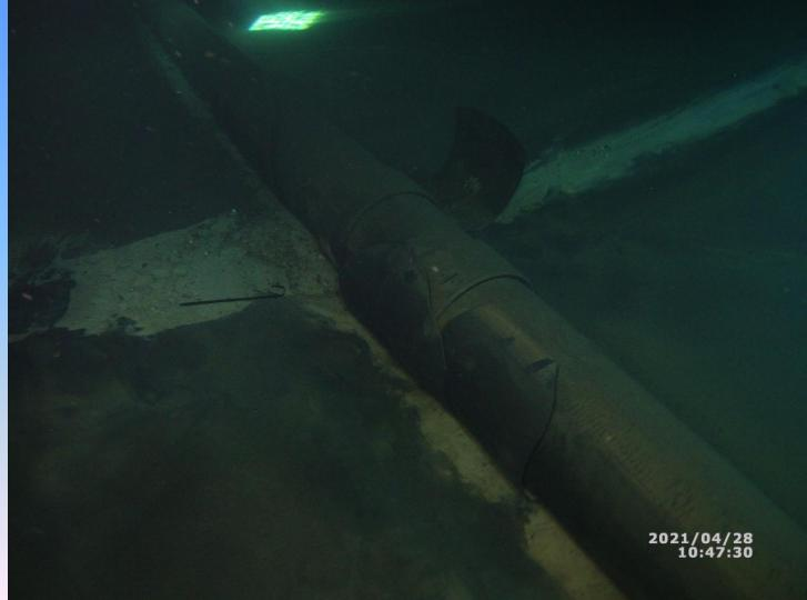
We opened the corners in order to remove the weight pipes from the floating liner.
