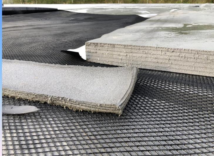
The insulation is so thin in some places, that the spikes from the fixation irons between the two lower layers is a threat to the floating liner.
