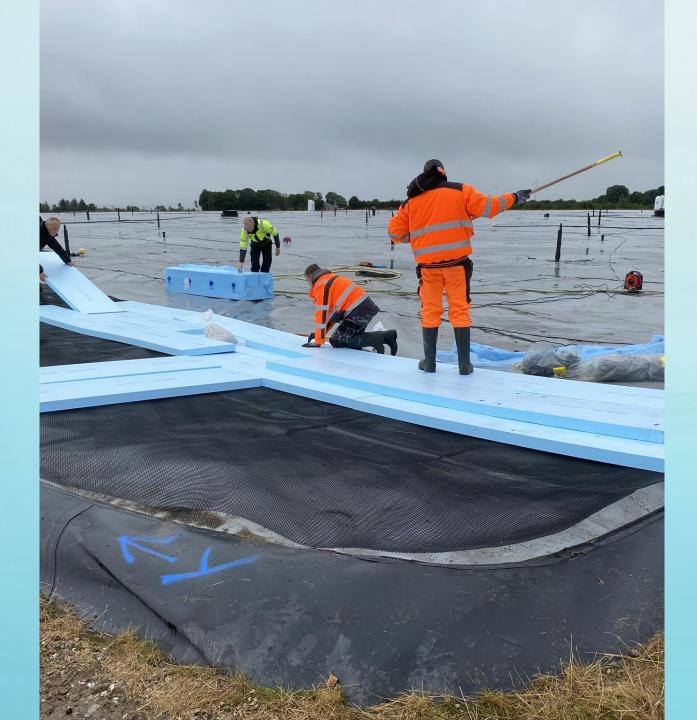
Plastic nails are tapped into the top insulation to hold the layers together.
