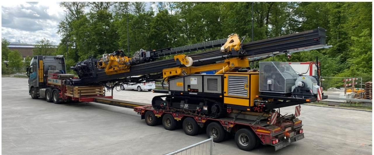
Figure 25: Delivery of rig on site.
