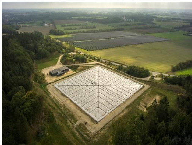
Figure 37: Aerial view of the PTES in Dronninglund.
