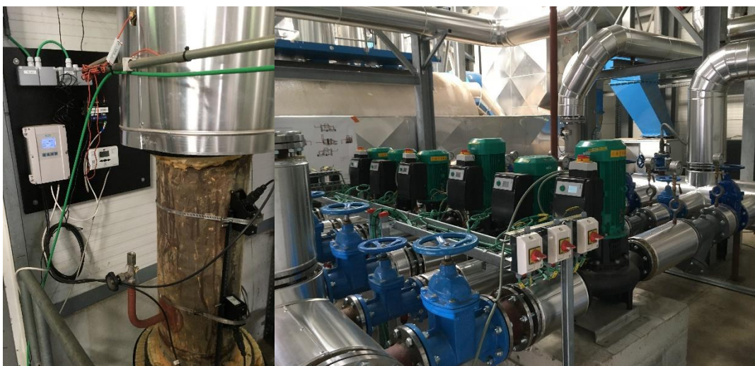
Figure 5: Left: Installation of an ultrasonic flowmeter, heat meter with IOT gateway on a DN250 DHN pipe. Right: New substation for the residential area.
